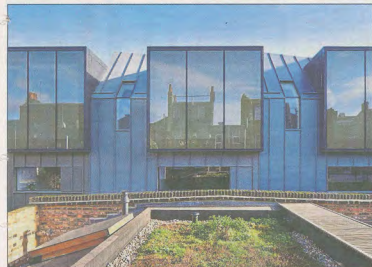
Super-light the flats, with big picture windows, are cantilevered in wood and the roofline is eye-catching
