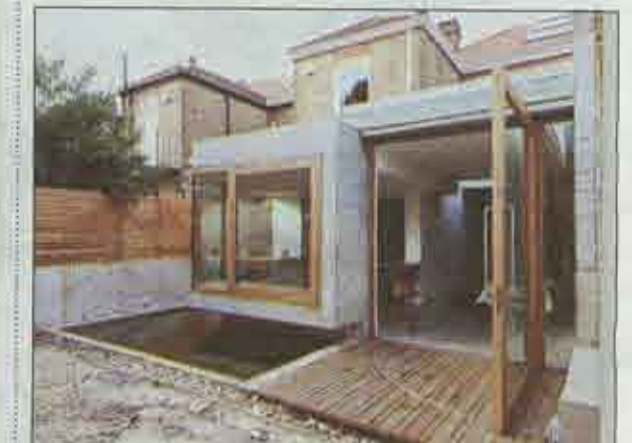
Above: exposed concrete is a feature of this transformation of a Victorian semi, Ruskin Park House, in Lambeth by AY Architects. A cantilevered bay window brings light to a new “family living” space. Cost: £325,000
